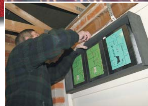
Upgrading an existing system.
